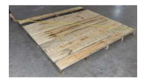
Step 3: Nail plastic weatherstrip to edge of floor on all four sides, with 30mm clouts, (approx 5 nails per side) ensuring top edge is flush with top of floor. This isn't required if shed is on a concrete base.
