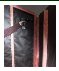
Step 6: Silicone edge of weatherboards on standing panel and nail on cedar beads with 5 x bead nails. (Refer to wall plan for correct beads).
